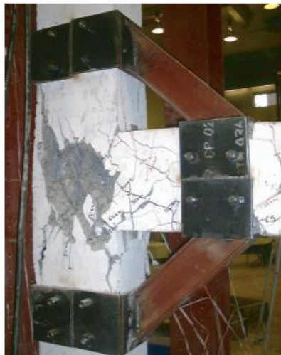
Figure 11 Steel braced column beam joint specimen with cracking formation [46].
